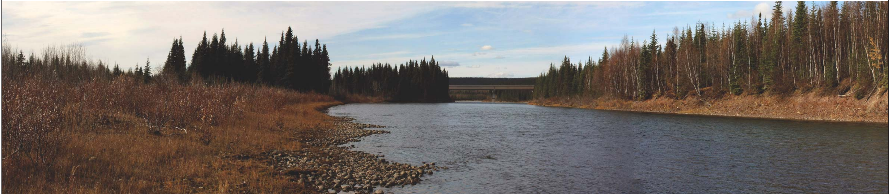
KOP 6 - Reed River 1 After Construction - Looking West (South Route)
