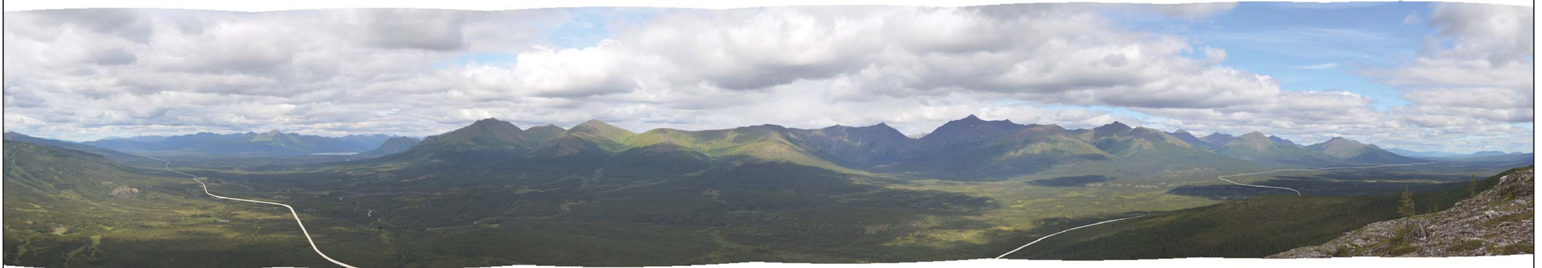
KOP 4 - ROW East Boundary After Construction - Looking North (North Route)
