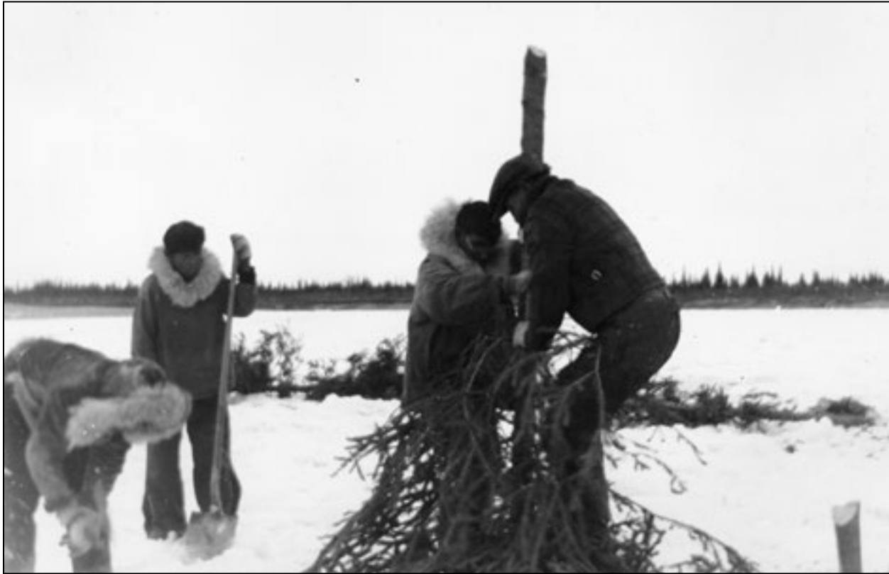
Plate 4-2.—Men building a fish trap under ice diversion for winter fishing.
