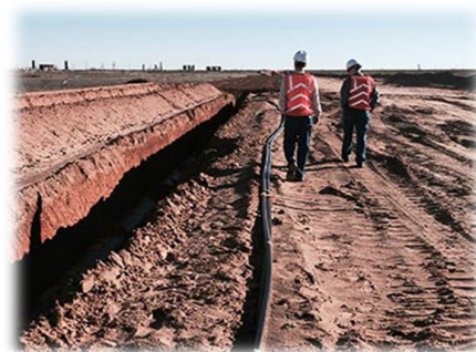
Figure 2: Typical fiber optic trench
